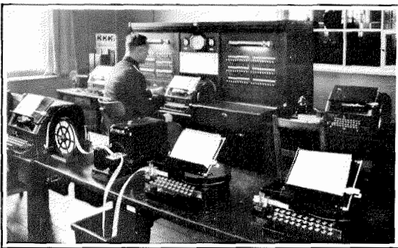
Figure 5—Automatic Transmitting Device at Berlin Police Headquarters
